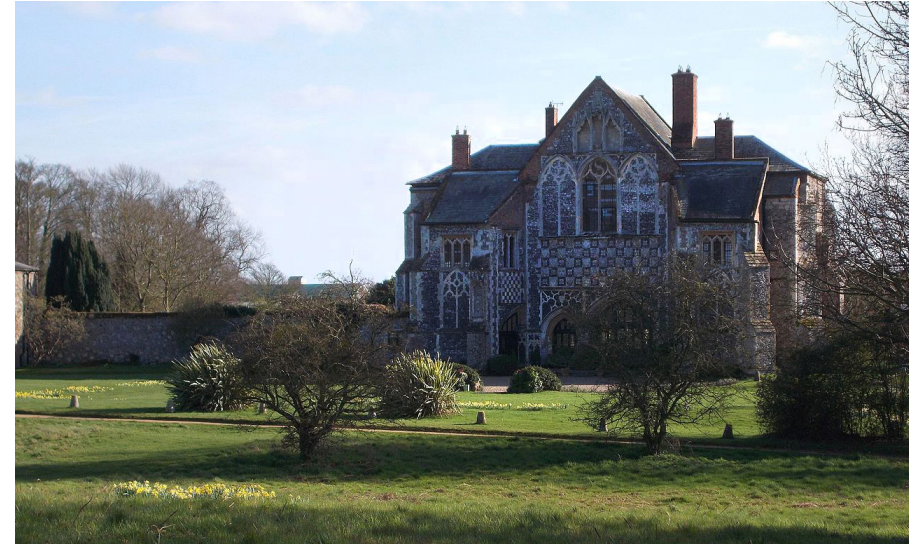
Fig 22: Butley Priory Gatehouse
