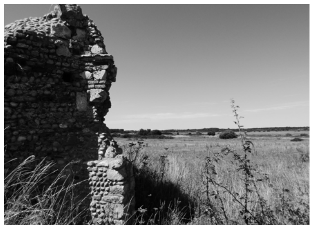
Fig 62: View towards Leiston from Eastbridge, Minsmere Chapel.
